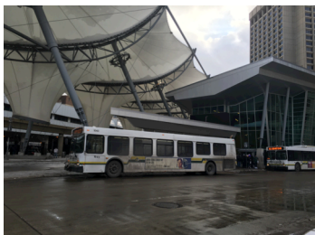
Figure 1. Exterior of Rosa Park Station and Buses
